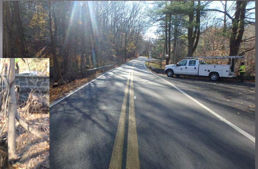
North Approach – Looking South
