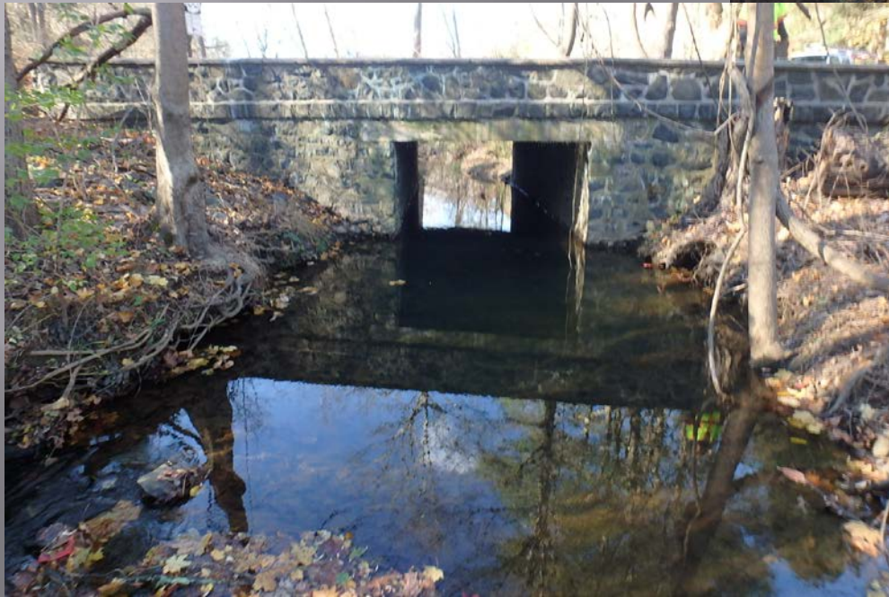
East Elevation View
