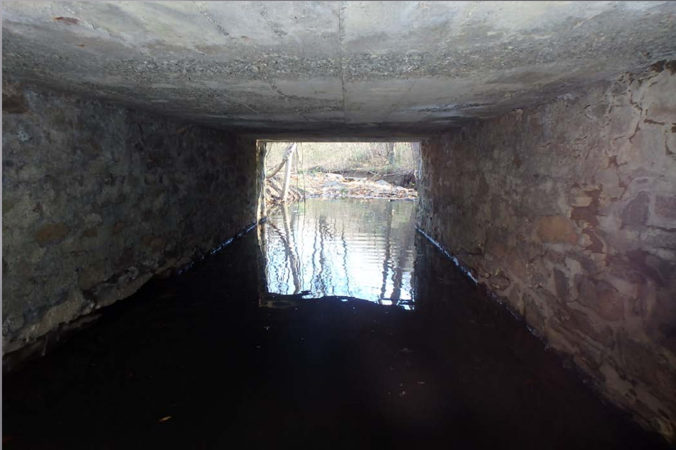
General View – Looking through bridge structure
